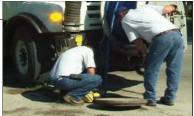
have been connected by residents over the years. Smoke testing is the most efficient way of identifying these illegal connections.
