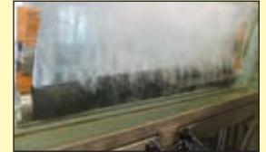
Diffuser with clogged membrane
