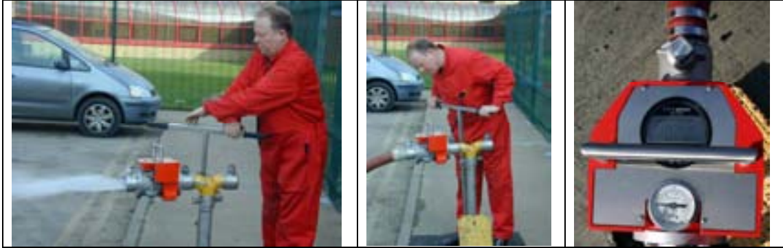
Picture 5: Testing an underground hydrant using a standpipe and an example of flow readout and residual pressure reading. Photos courtesy of Essex County Fire and Rescue Service and Laois Fire Service.
